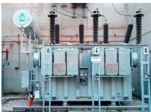
Novi energetski transformator T1
