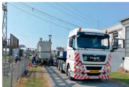
Istovar transformatora T2
