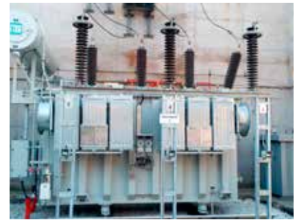
Novi energetska transformator T2
