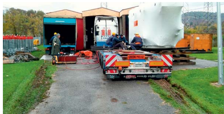
TS ZVORNIK - istovar transformatora T20 110/35/10 kV - 20 MVA
